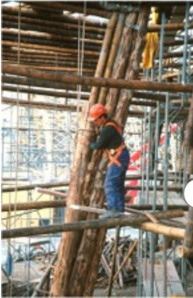
STAGE 3: Installation of columns and guadua support rings – reinforcement of roof.
