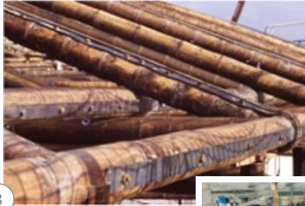
STAGE 4: Construction of tuss, beams and diagonal support.
