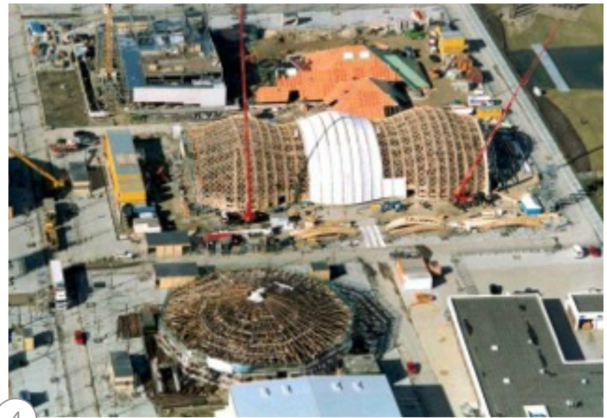
STAGE 4: Construction of tuss, beams and diagonal support.
