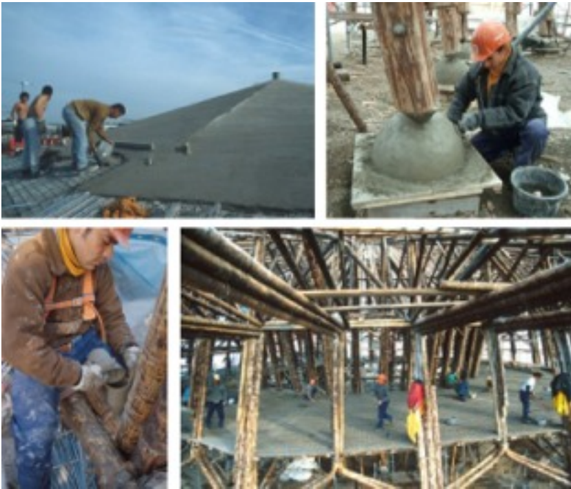
From left up to right down: Roof, Footings, Guadua chambers and Mezzanine.
